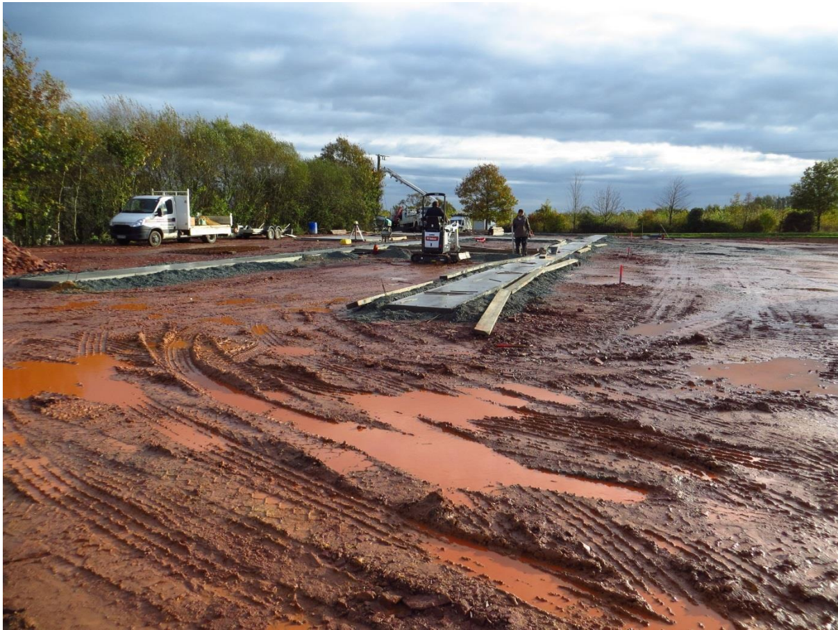
Figure 16. The construction of new buildings as part of Project Vegepole
