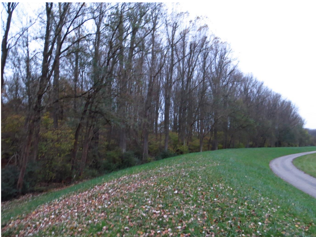
Figure 3. Wet woodland polder in Speyer, protecting the airport and chemical industry from flooding, with a recreational route alongside
