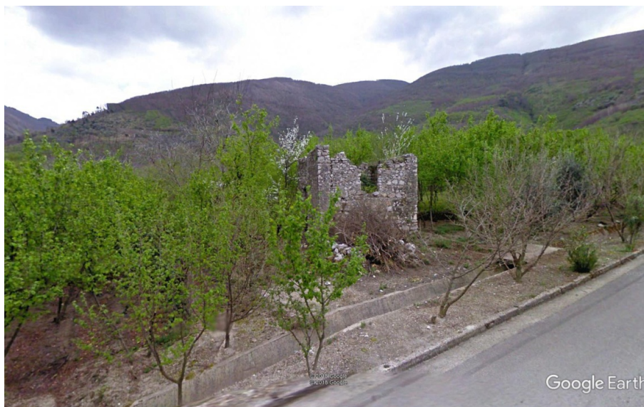
Figure C.45 Rural building of Quindici (AV) [source: Google Earth]
