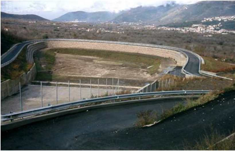
Figure C.13 Pietra di Valle Detention Basin of Quindici (AV) Municipality
